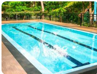
Medirigiriya Project Needs International School
